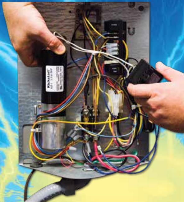
A proper starting device can extend the life of your compressor, by having a quicker, more efficient start.
