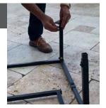
For concrete pad application, recommend to use Tapcon ¼" x 2½" Phillips countersunk #24585. When inadequate pad clearance is an issue, consider two lock locations on either side of the pad. Dig holes to fill with Sakcrete mix and water before mounting foot brackets securely onto the filled liquid concrete.
